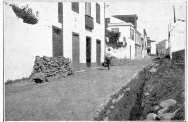
FIG. 8.—FISSURE CAUSED BY EARTHQUAKE.
