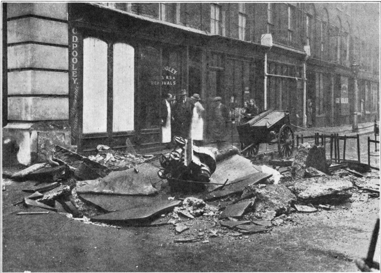
FIG. 2.—OUTSIDE MANHOLE WHERE FIRST EXPLOSION TOOK PLACE.
