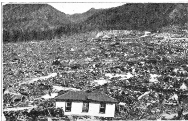
FIG. 4.—MATARITAKI SLIP. VALLEY FILLED TO DEPTH OF 80 FEET. ONE HOUSE BURIED AND 4 PERSONS PERISHED. HOUSE IN FOREGROUND IS TOP STOREY OF ANOTHER HOUSE AFTER MOVING \frac{1}{2} MILE.
