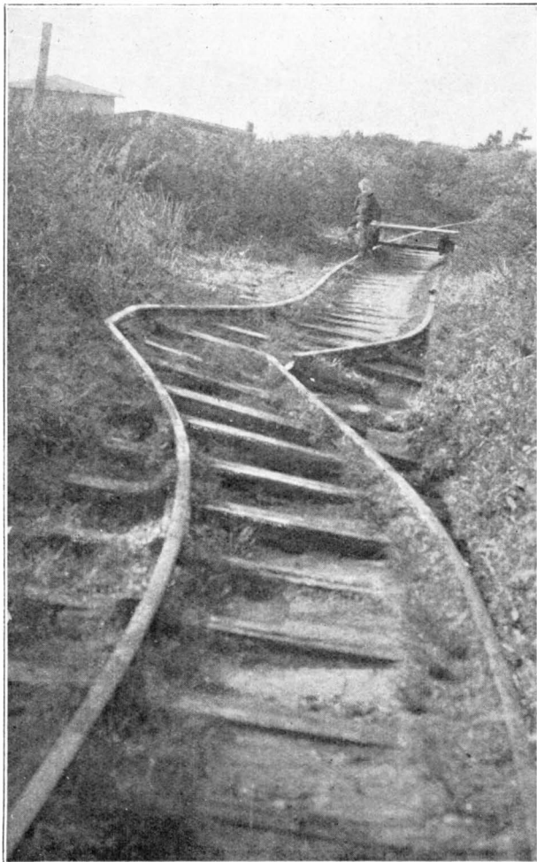
FIG. 9.—WESTPORT. HARBOUR BOARD'S RAILWAY LINE.
