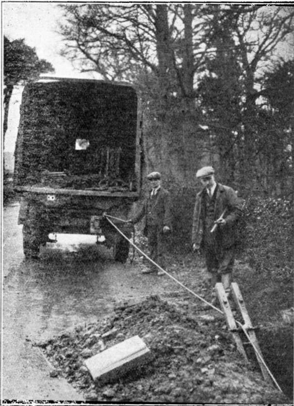
FIG. 3.—DRAW-ROPE HITCHED TO LORRY.
