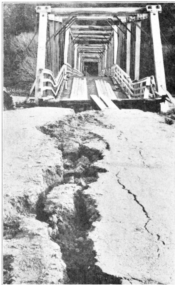
FIG. 3.—MURCHISON. MATAKITAKI BRIDGE AND APPROACH.
