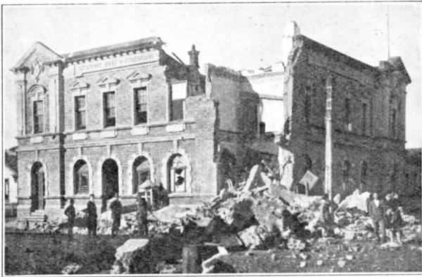
FIG. 8.—WESTPORT. POST AND TELEGRAPH OFFICE.
