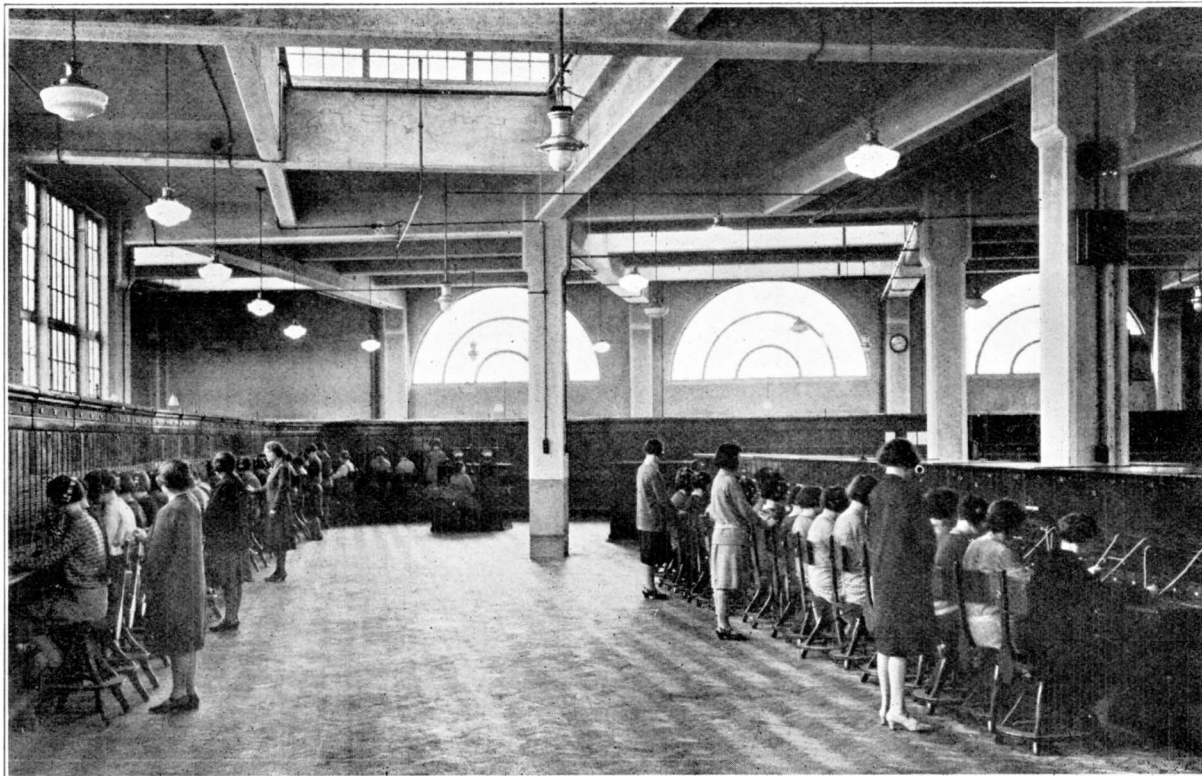
FIG. 2.—VIEW OF MANUAL SWITCHROOM.
