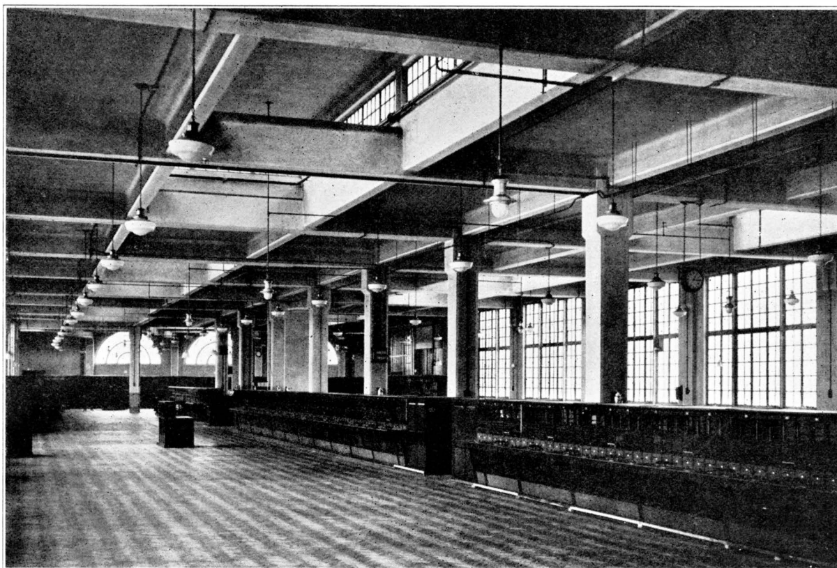
FIG. 3.—ANOTHER VIEW OF MANUAL SWITCHROOM.
