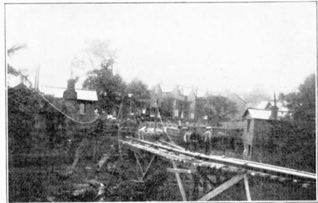
TEMPORARY BRIDGE TO CARRY WATER MAINS, BUILT BY THE R.E.'S.
