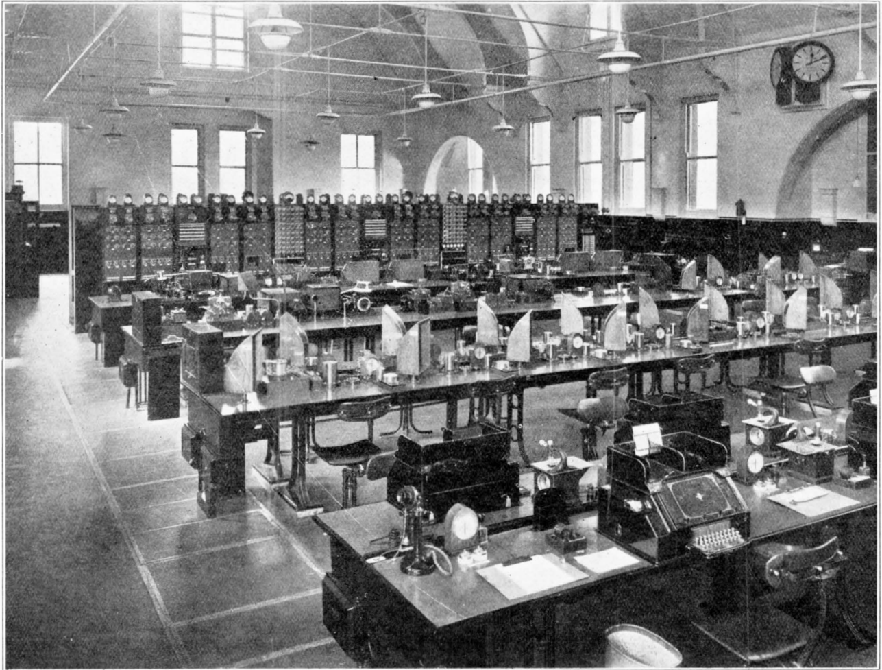
FIG. 4.—PART OF INSTRUMENT ROOM, SHOWING THREE SECTIONS OF BAYS IN BACKGROUND.
