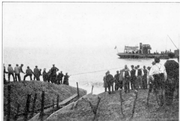
FIG. 2.—PULLING END ASHORE FROM " KATHARINE."
