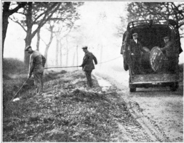
FIG. 3.—LAYING THE CABLE.
