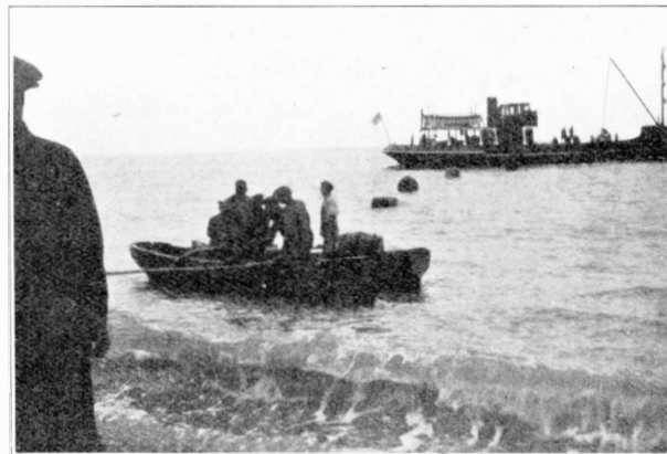
FIG. 3.—LANDING THE END.
