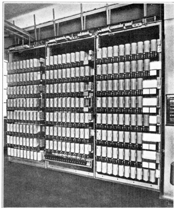
FIG. 5.—COMMON CONTROL SELECTORS AT BISHOPSGATE.
