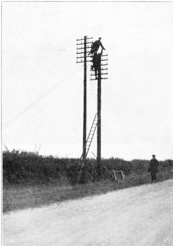
FIG. 4.—CHANGING OVER THE WIRES.
