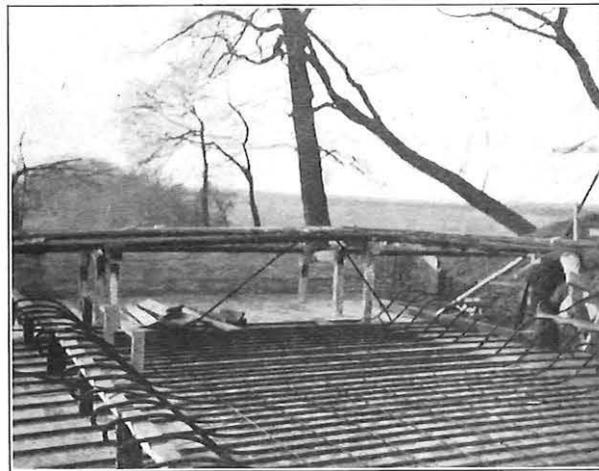
FIG. 1.—PIPES SUPPORTED ON SHUTTERING.
