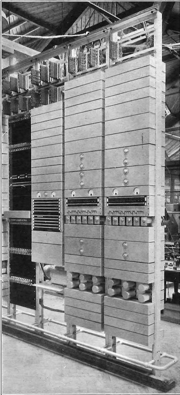
FIG. 8.—TYPICAL 12-CHANNEL EQUIPMENT.
