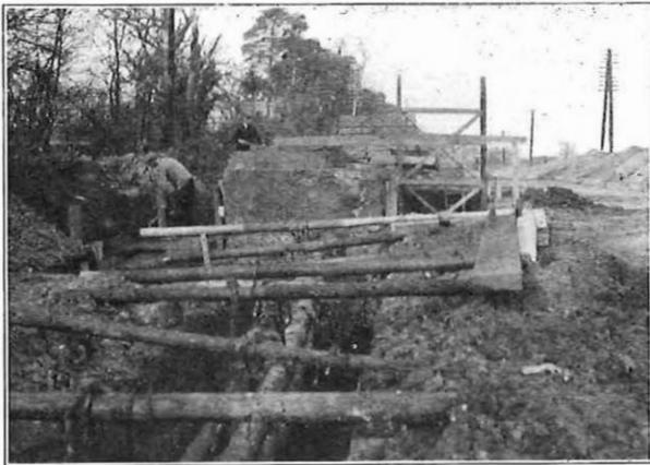
FIG. 1.—MANHOLE READY FOR LOWERING.
