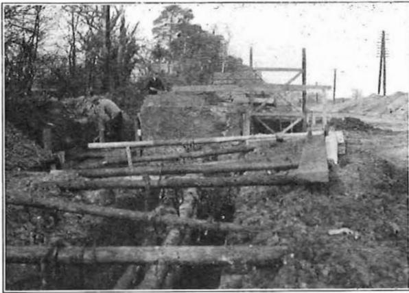
FIG. 1.—MANHOLE READY FOR LOWERING.
