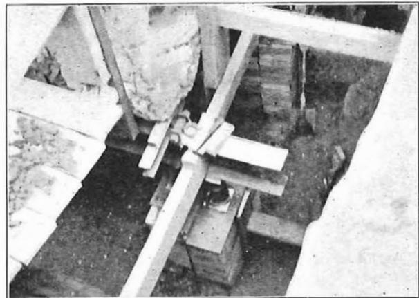
FIG. 2.—METHOD OF SUPPORTING MANHOLE.
