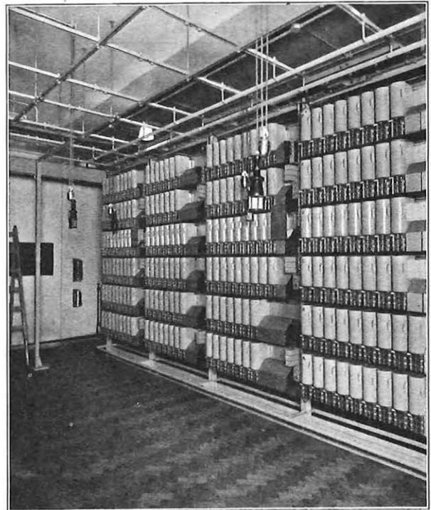
FIG. 5.—FINAL SELECTORS, CENTRAL EXCHANGE.
