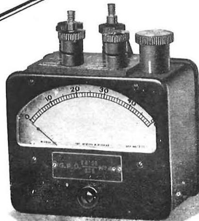
This instrument was designed by us for the British Post Office, and is now a standard instrument in that service and the majority of the Dominion and Colonial P. & T. Services, with the Post Office designation "Detector" No. 4.
