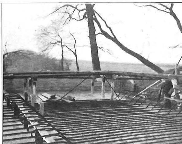
FIG. 1.—PIPES SUPPORTED ON SHUTTERING.
