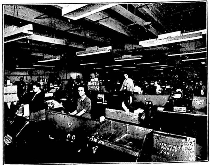
FIG. 8.—TYPICAL FLUORESCENT LIGHTING INSTALLATION.
