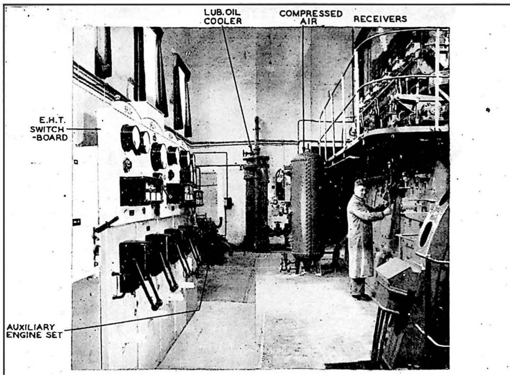
FIG. 3. GENERAL VIEW OF ENGINE AND E.H.T. SWITCHBOARD.
