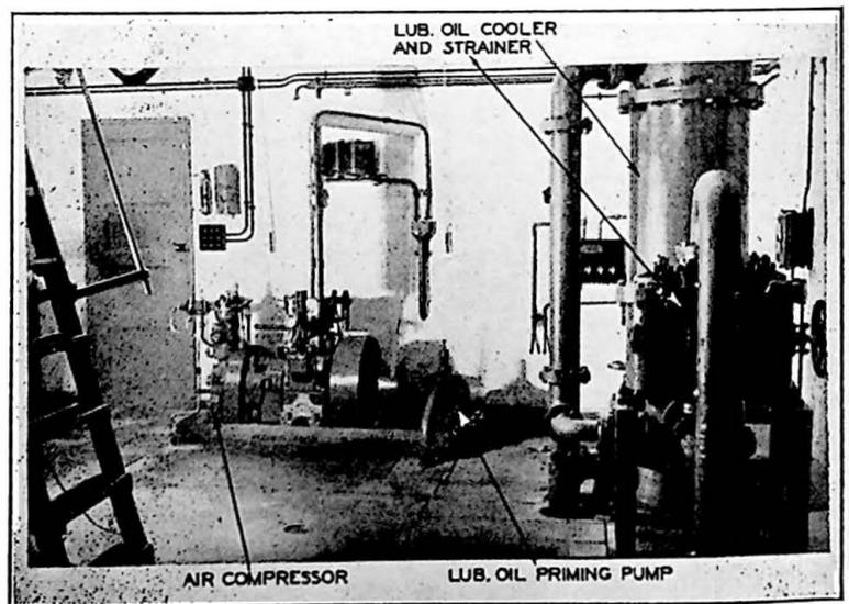
FIG. 5. AUXILIARY EQUIPMENT.
