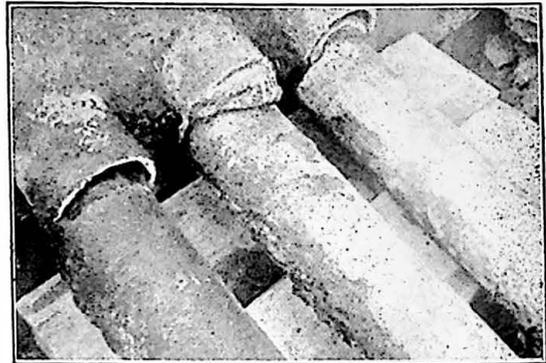
was very loose and waterlogged, and it would appear that the trouble was due to faulty consolidation after the bridge was rebuilt, or entry of water under the road, so causing the road foundation to become loose, or possibly a combination of both. The pipes entering the bridge structure were thus virtually left with no underneath support, and the continual heavy traffic on the main road resulted in the fractures.
