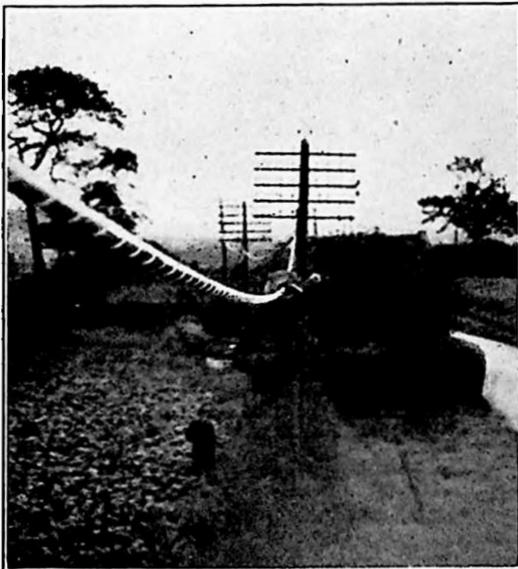
FIG. 4. CABLE SPAN PARTLY COMPLETED.
