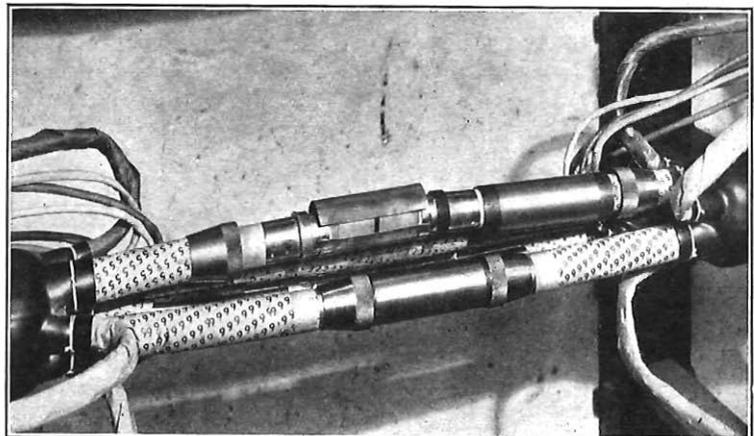
FIG. 5.—CONSTRUCTION OF JOINTS IN 0.975 INCH TUBES.
