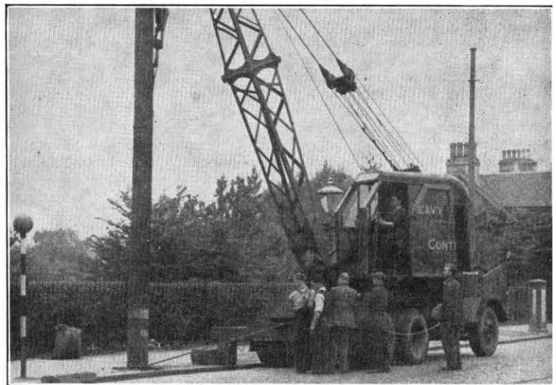
FIG. 2.—LIFTING THE POLE.
