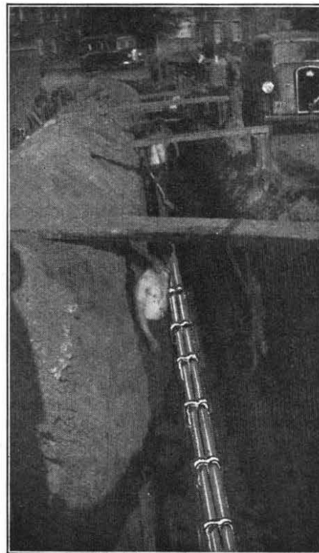
GENERAL VIEW OF THE EXCAVATION.
