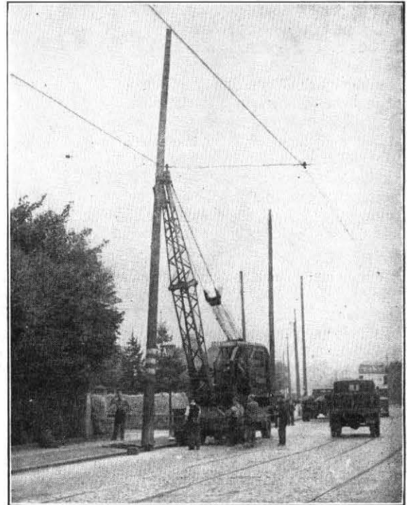
FIG. 1.—POSITIONING THE CRANE.
