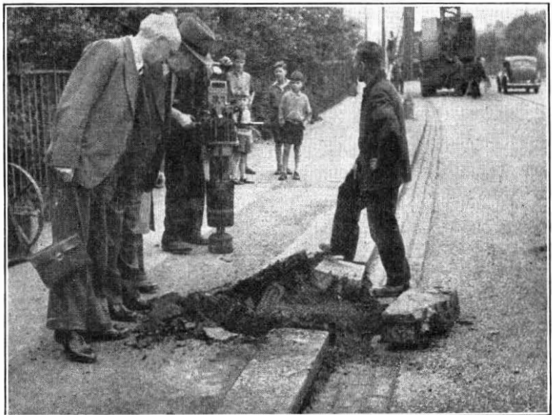
FIG. 4.—DISTURBANCE OF FOOTWAY—THE WORST CASE.
