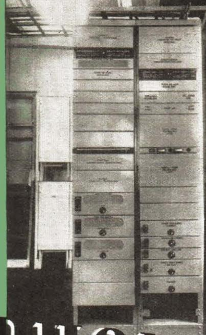
Above—12-Circuit open-wire equipment in the trunk telephone system of Turkey.
