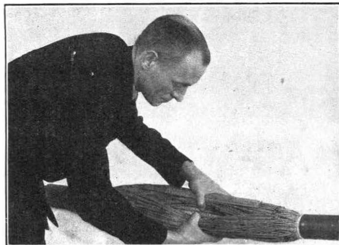
FIG. 2.—BARREL TYPE JOINT COMPLETED; SHOWING LIMITED ACCESS TO COAXIAL PAIRS.
