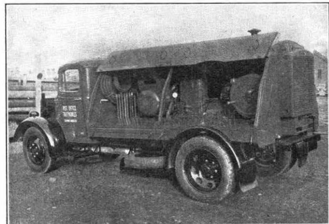
FIG. 2.—SELF-MOBILE AIR-COMPRESSOR WITH SIDE CANOPY OPEN.
