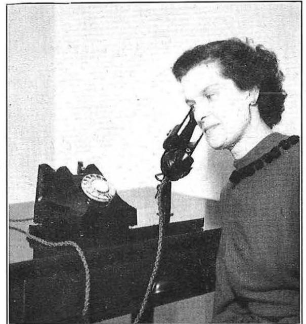
METHOD OF USING HANDSET IN ADJUSTABLE CRADLE.
