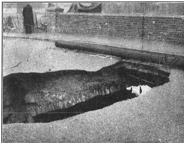
HOLE IN BRIDGE AT HADLOW, SHOWING TEMPORARY SUPPORT FOR ONE POST OFFICE CABLE.
