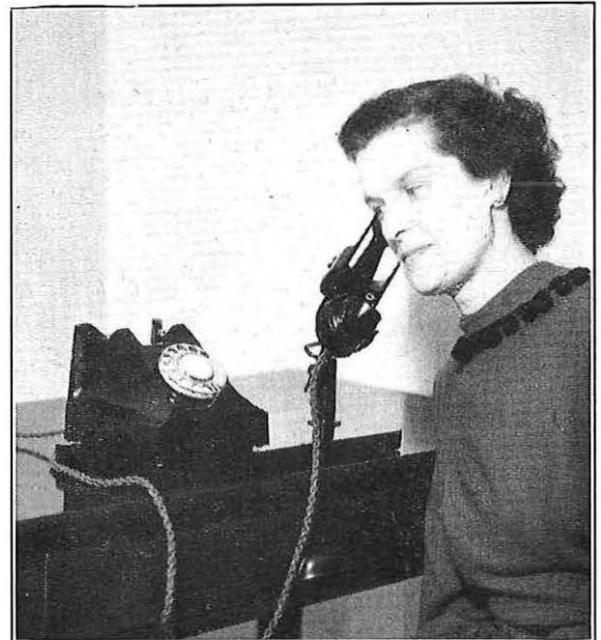
METHOD OF USING HANDSET IN ADJUSTABLE CRADLE.
