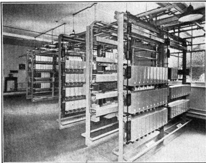
FIG. 21.—TYPICAL 500-LINE INSTALLATION OF P.A.B.X. No. 3.
