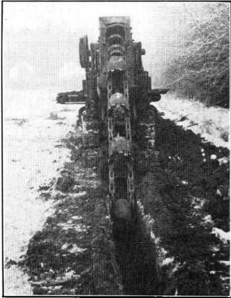
FIG. 13.—TRENCH EXCAVATOR.
