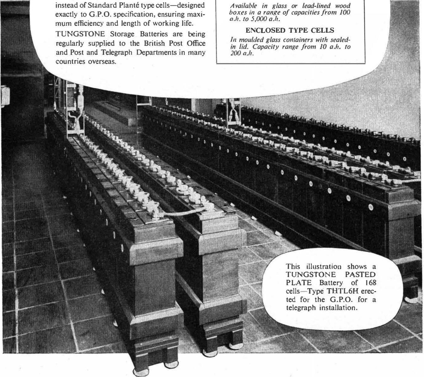
This illustration shows a TUNGSTONE PASTED PLATE Battery of 168 cells—Type THTL6H erected for the G.P.O. for a telegraph installation.
