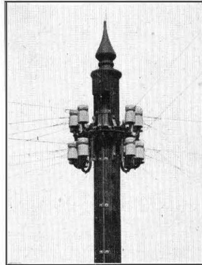
FIG. 5.—THE TOP OF A RING-TYPE DISTRIBUTION POLE.
