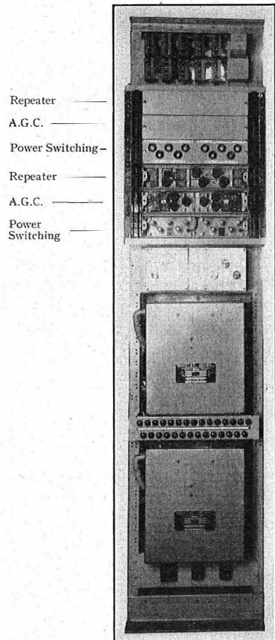
FIG. 14.—LINE EQUIPMENT FOR POWER FEEDING STATION.
