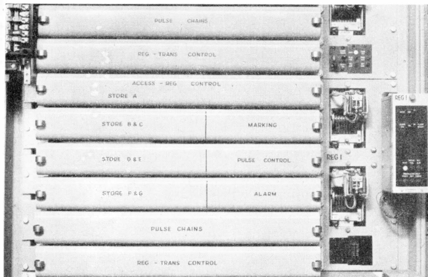
FIG. 2—INCOMING ELECTROMECHANICAL REGISTER FOR DIRECTOR AREAS
