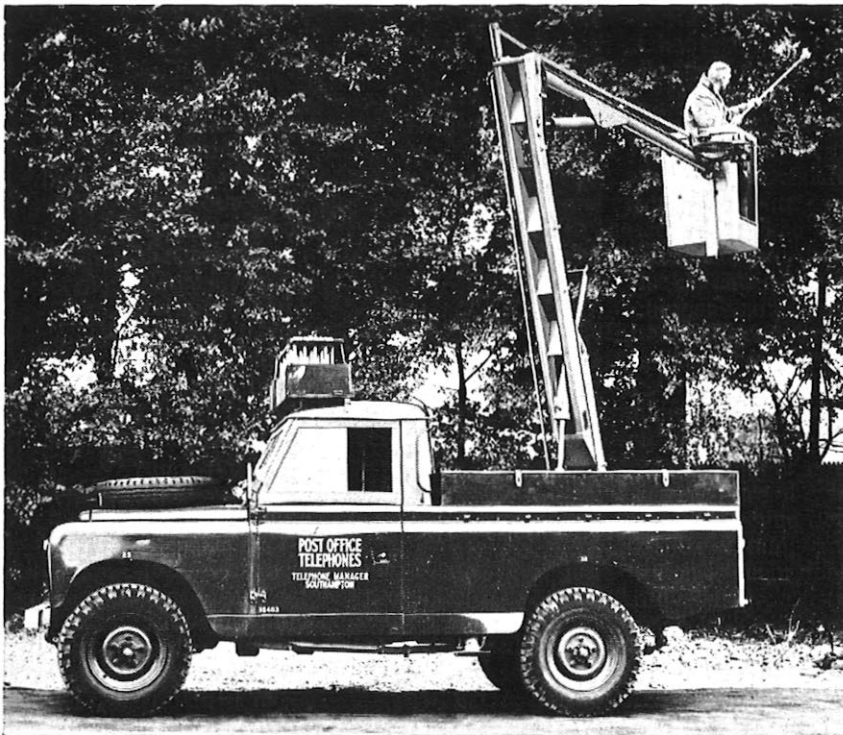
FIG. 2—ELEVATING PLATFORM IN USE
