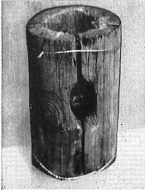
THE SECTION OF POLE DAMAGED BY WOODPECKERS
