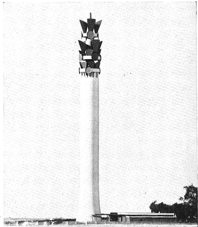
FIG. 11—MODEL OF A MAIN-ROUTE MICROWAVE RADIO-RELAY REPEATER STATION WITH A CONCRETE TOWER
