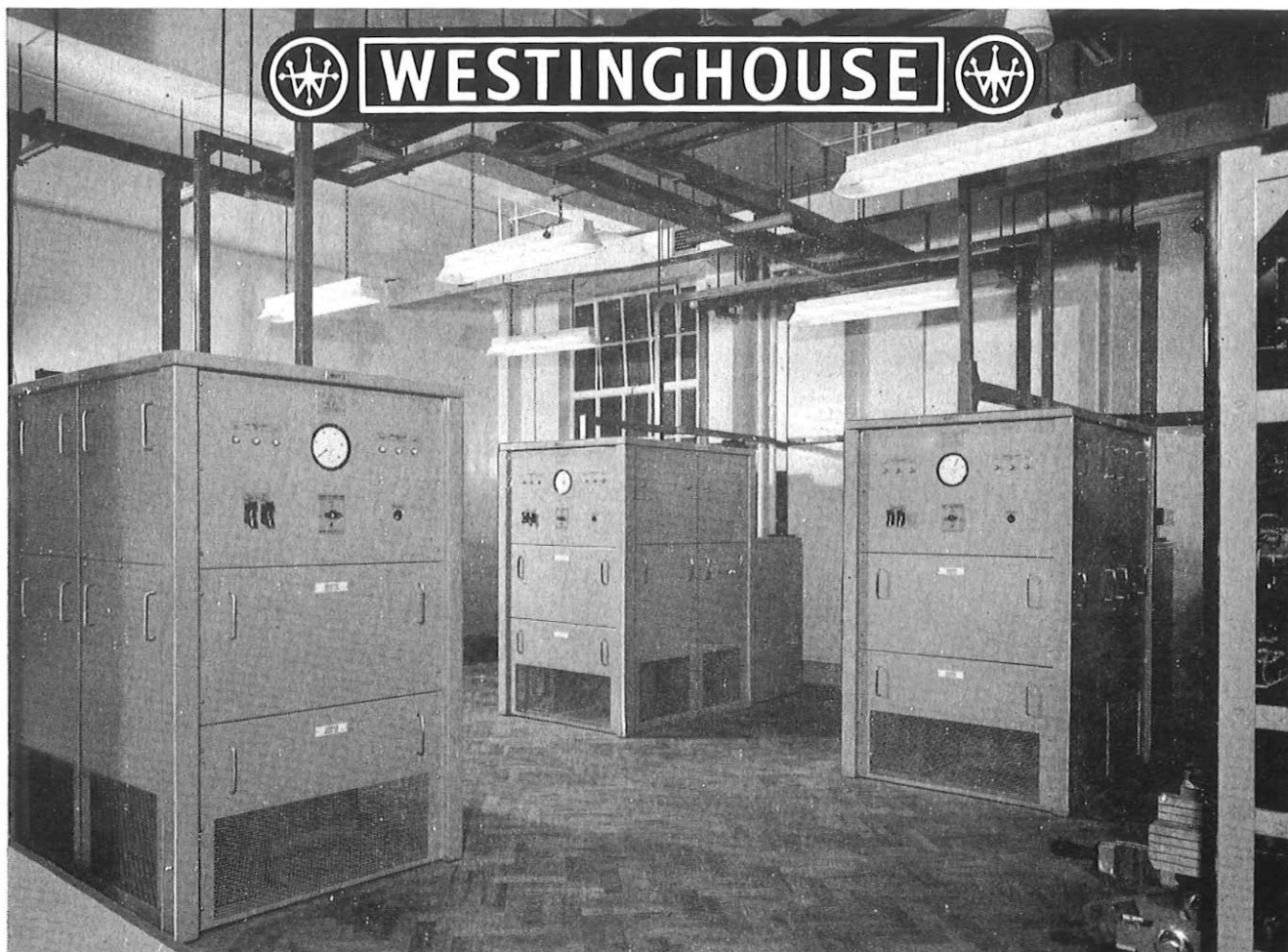
Mechanically regulated germanium rectifier equipments at the B.P.O. Whitehall telephone exchange
