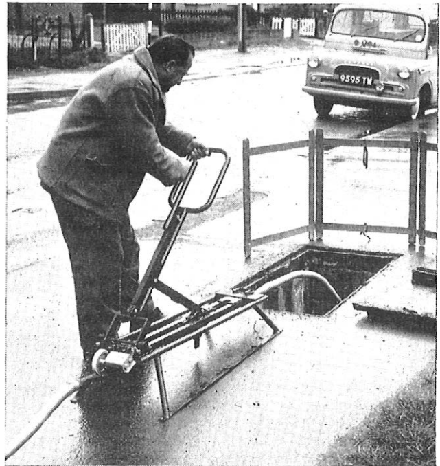
FIG. 3—MACHINE SET UP FOR RODDING A DUCT
