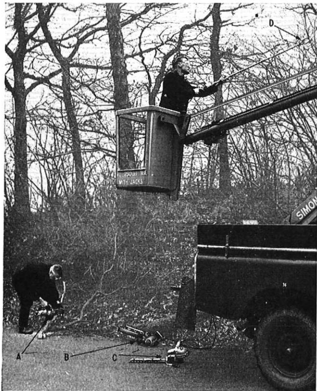
A—Five-inch saw. B—Twelve-inch saw. C—Hedge-cutter. D—Pruner FIG. 2—TREE-CUTTING TOOLS
