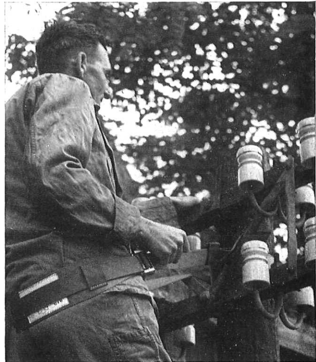
FIG. 4—LENGTHENING THE LOOP OF THE POLE BELT
