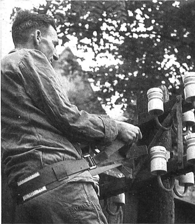
FIG. 3—SHORTENING THE LOOP OF THE POLE BELT
