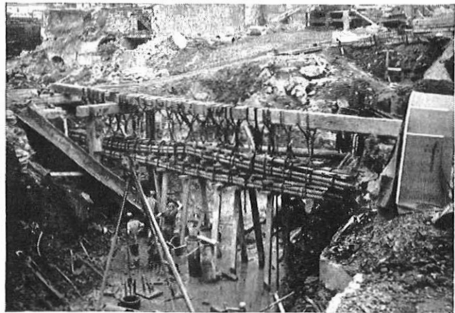
CABLES SUSPENDED OVER ROAD WORKS AT NEWCASTLE
