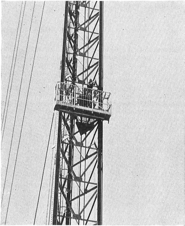
FIG. 9—SKIP IN POSITION ON FACE OF MAST
