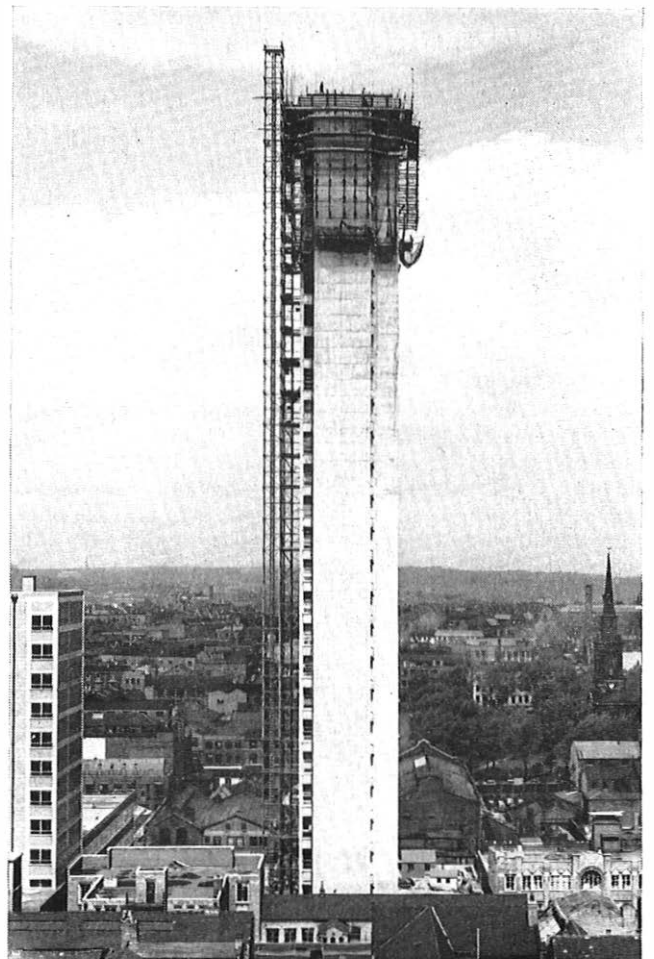
FIG. 3—TOWER UNDER CONSTRUCTION
