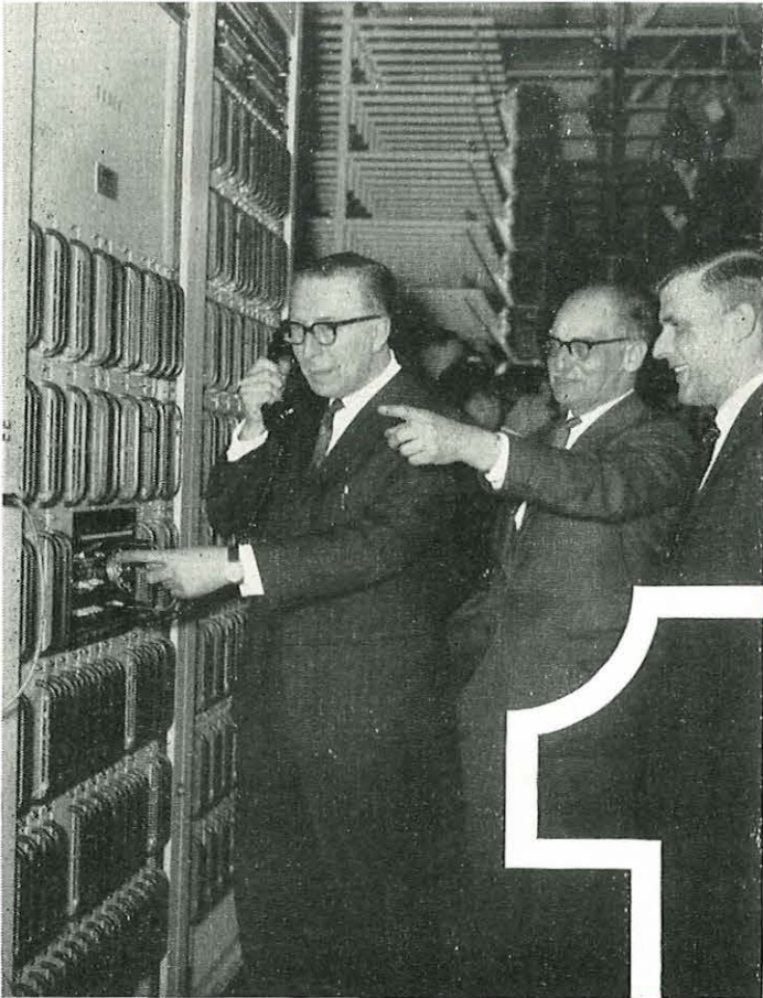
Mr. J. A. Lawrence, Senior Staff Engineer T.P.E. Branch of the G.P.O. tries out the electronic exchange equipment at Leamington Spa following its switch into public service.
