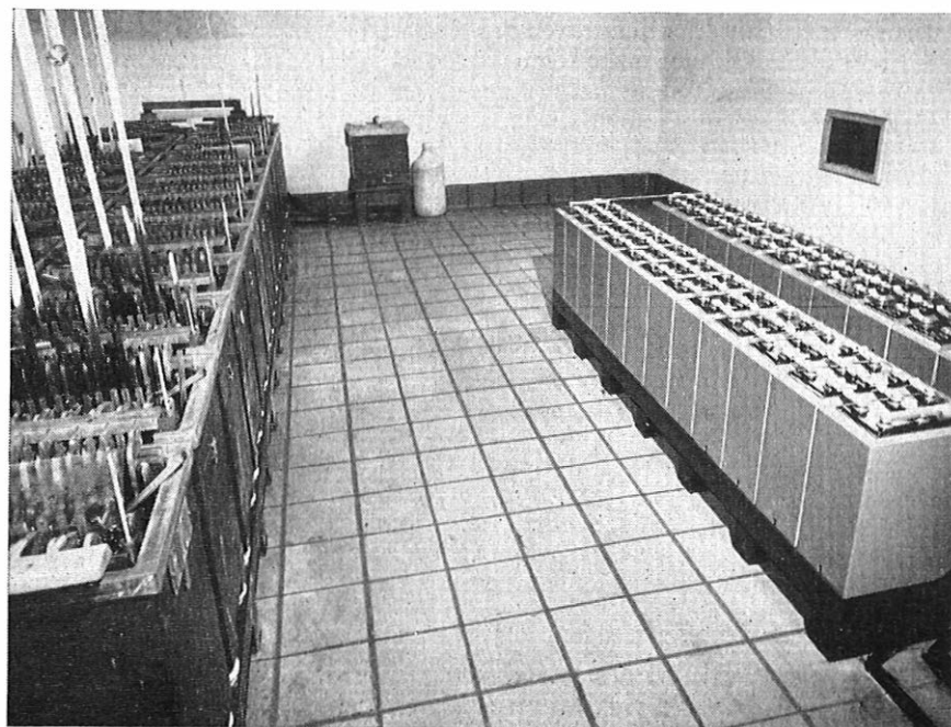
Wooden laths, inserted to prevent contact between distorted positive plates and the negative plates can be seen in the old battery on the left-hand side
