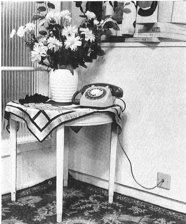
FIG. 2—TELEPHONE TERMINATION INSIDE HOUSE
