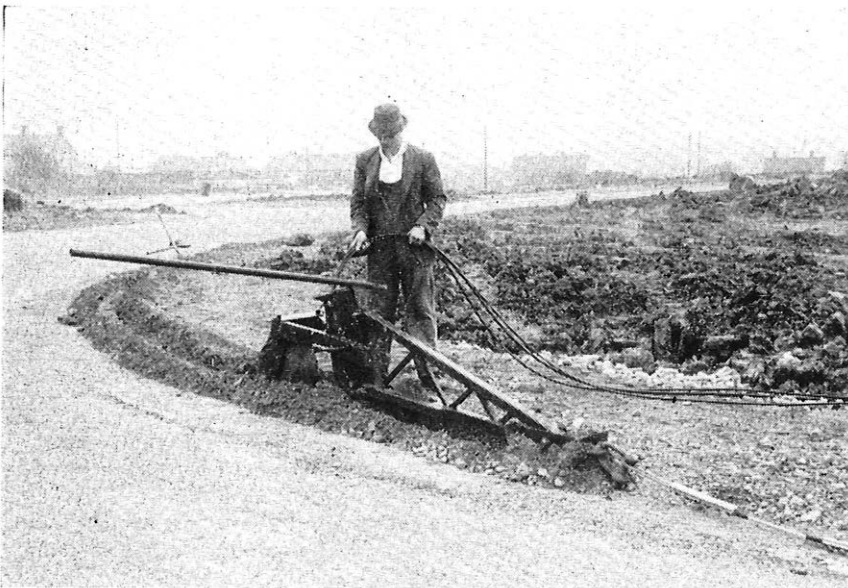
FIG. 5—POST OFFICE FOOTPATH CABLES BEING LAID BY MOLEPLOUGH BEFORE BUILDING MATERIALS ARE DEPOSITED ON THE FOOTPATH
