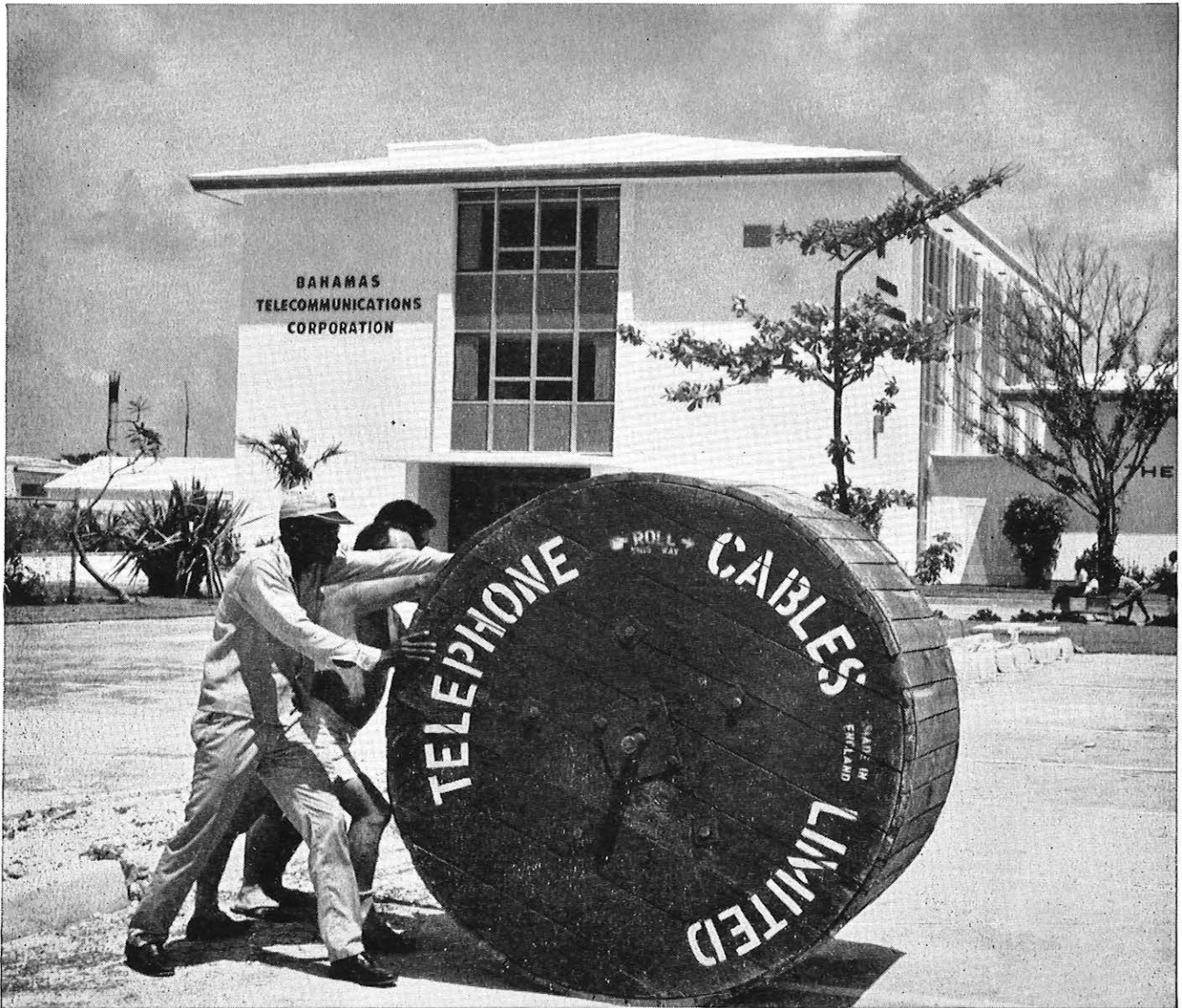
TCL cables being laid for the Bahamas Telecommunications Corporation
