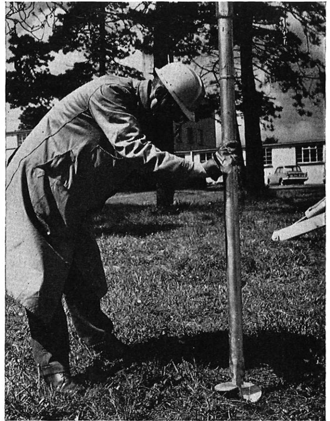
FIG. 6—SCREW-IN STAY ANCHOR AND ADAPTOR BEING STARTED INTO THE GROUND
