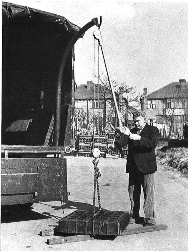
FIG. 1—EARLY-TYPE JIB BEING USED TO HANDLE HEAVY MANHOLE COVER
