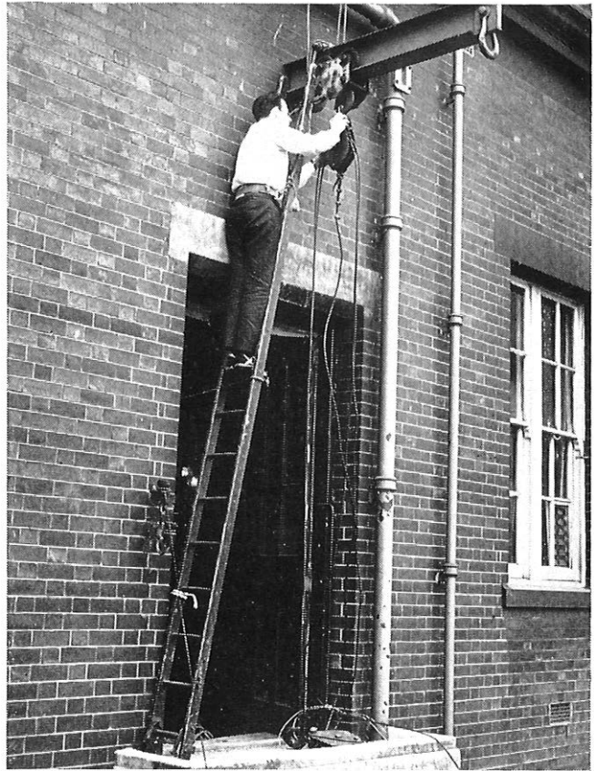
ATTACHING THE PULLEY TO THE CATHEAD
