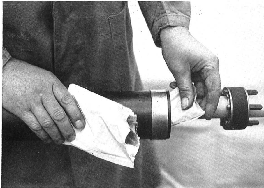
INSERTING SILICA-GEL SACHET INTO SLEEVE OF CABLE JOINT
