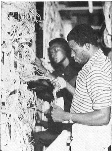
Wiring a crossbar exchange during installation in Nigeria.
