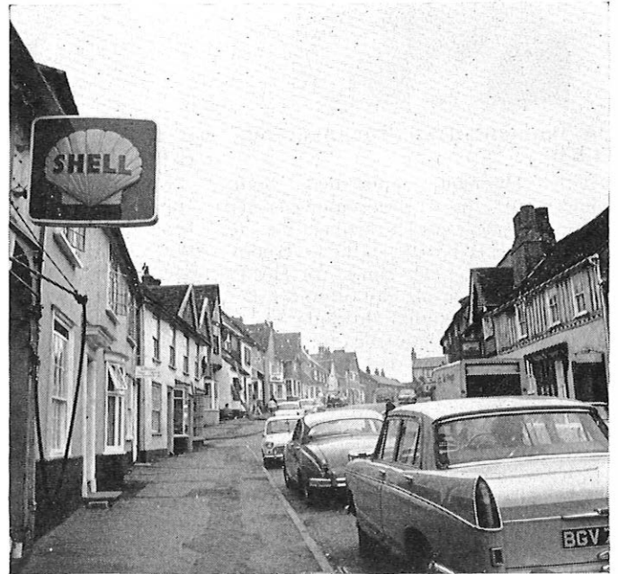
The same scene after the work was completed
