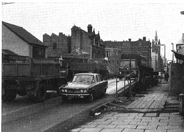
The girder bridge over the work
