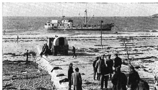
The Jersey end of the cable being taken ashore from the Cables ship Poolster.
