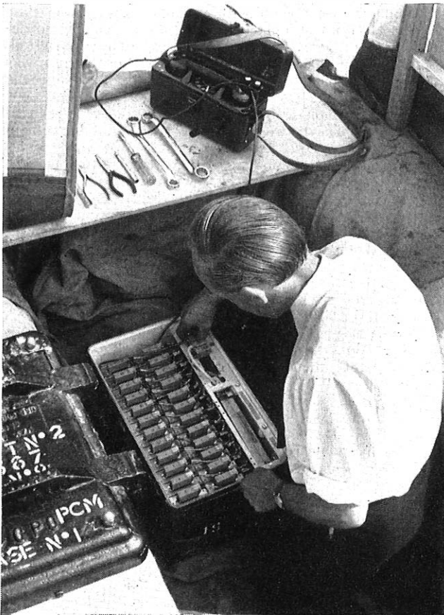
Installing a repeater
