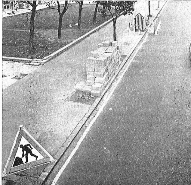
FIG. 2—Layout of guarding equipment: plant in the footway; daytime working
