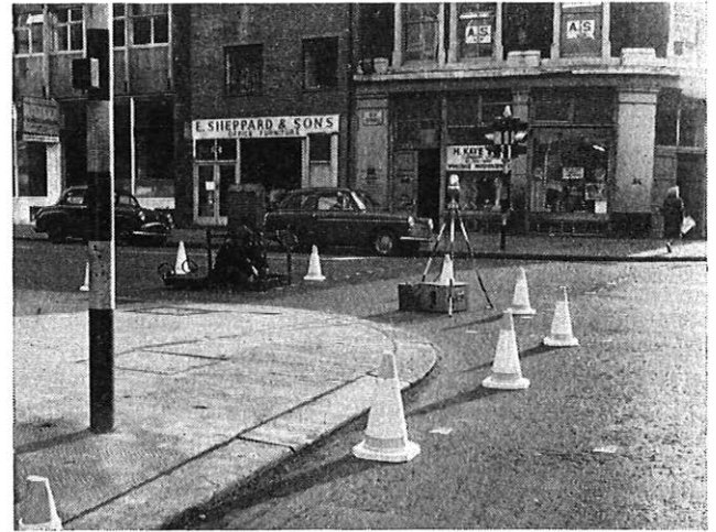
(b) Full view of the obstruction with the guarding arrangements
