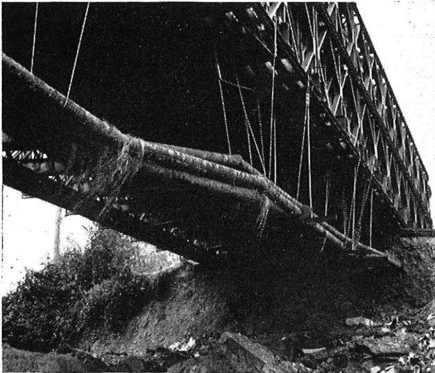
Steel pipes supported by the Bailey bridge
