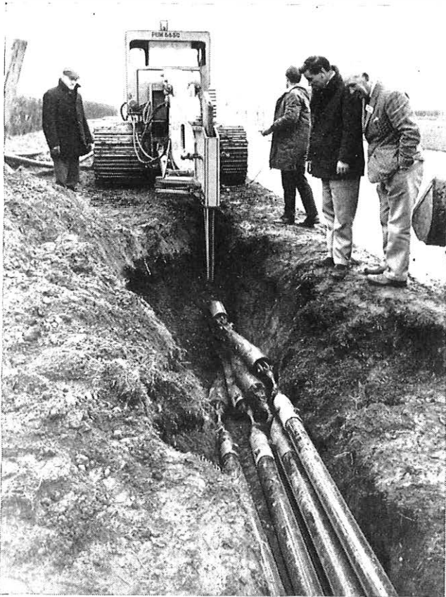
Badger Minor machine showing method of connexion to p.v.c. pipes
