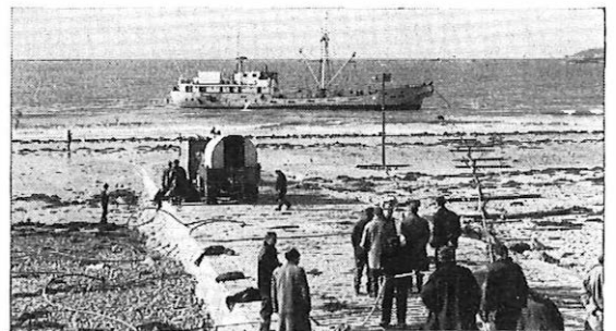
The Jersey end of the cable being taken ashore from the Cables ship Poolster.
