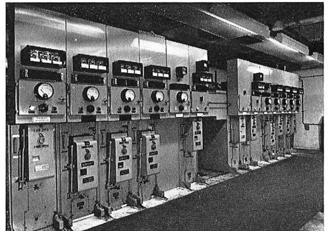
Fig. 1—Thirteen-panel high-voltage board in Mount Pleasant sub-station
