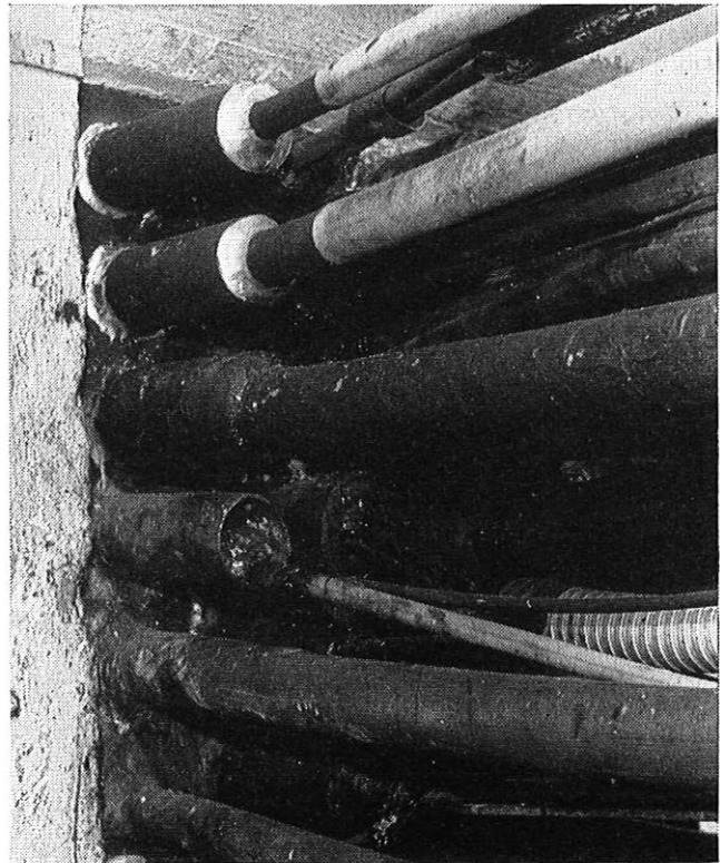
FIG. 1—The old duct-seal
