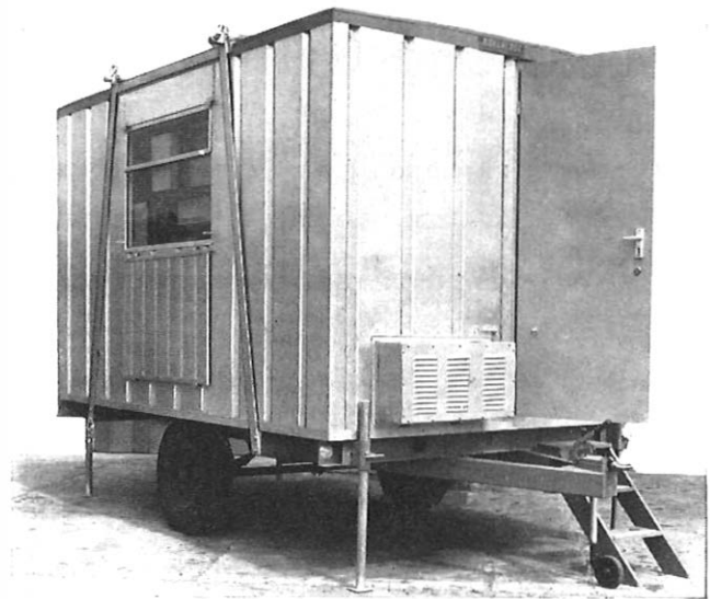
FIG. 6—External view of trailer caravan showing air conditioner intake
