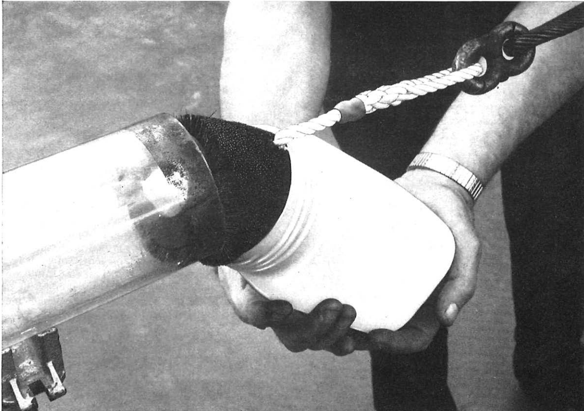
FIG. 5—Lubricating brush entering duct
