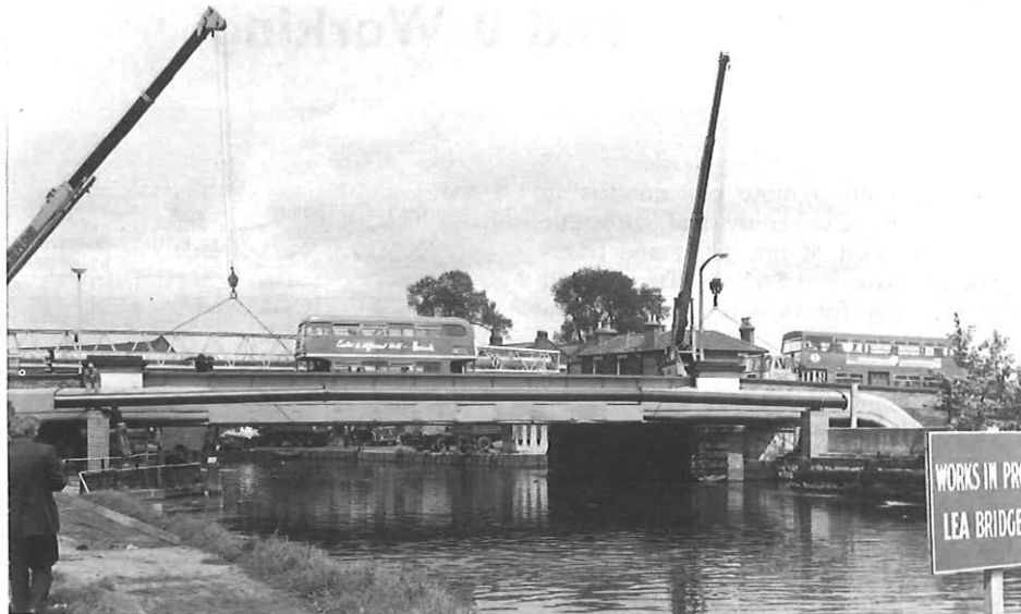
FIG. 1—The main span over the River Lea
