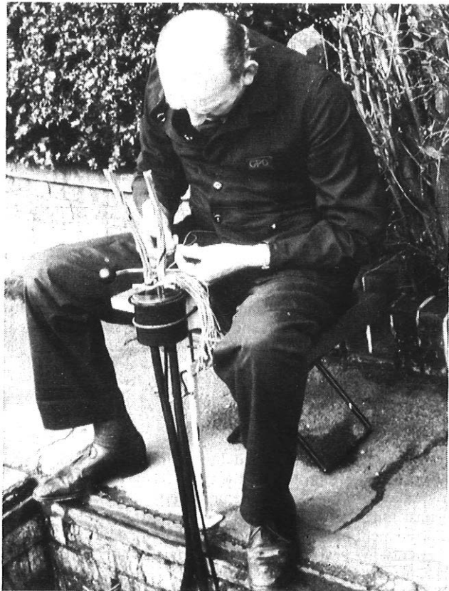
FIG. 9—Sleeve No. 31A with a jointing jig
