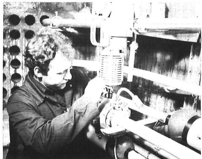
FIG. 11—Injection welding of sheath closure in progress
