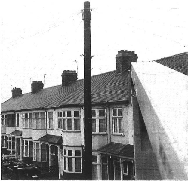
FIG. 12—A modern wood distribution pole
