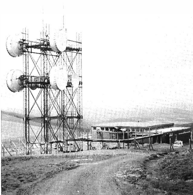
FIG. 15—Tower No. 5A
