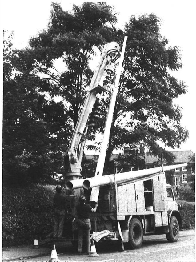
FIG. 13—Pole-Erection Unit erecting a hollow pole
