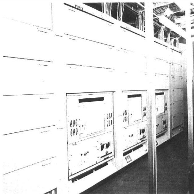
FIG. 9—System X large processor utility
