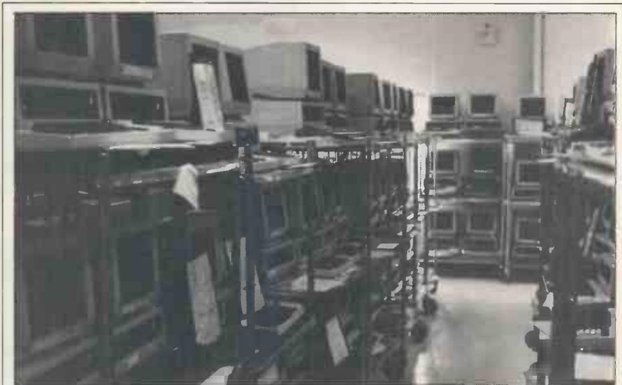
A roomful of Victors and Sirius is undergoing soak testing and generating an amazing amount of heat at the same time...
