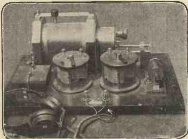
A very neat inductively coupled crystal receiver, using two condensers for tuning purposes.
