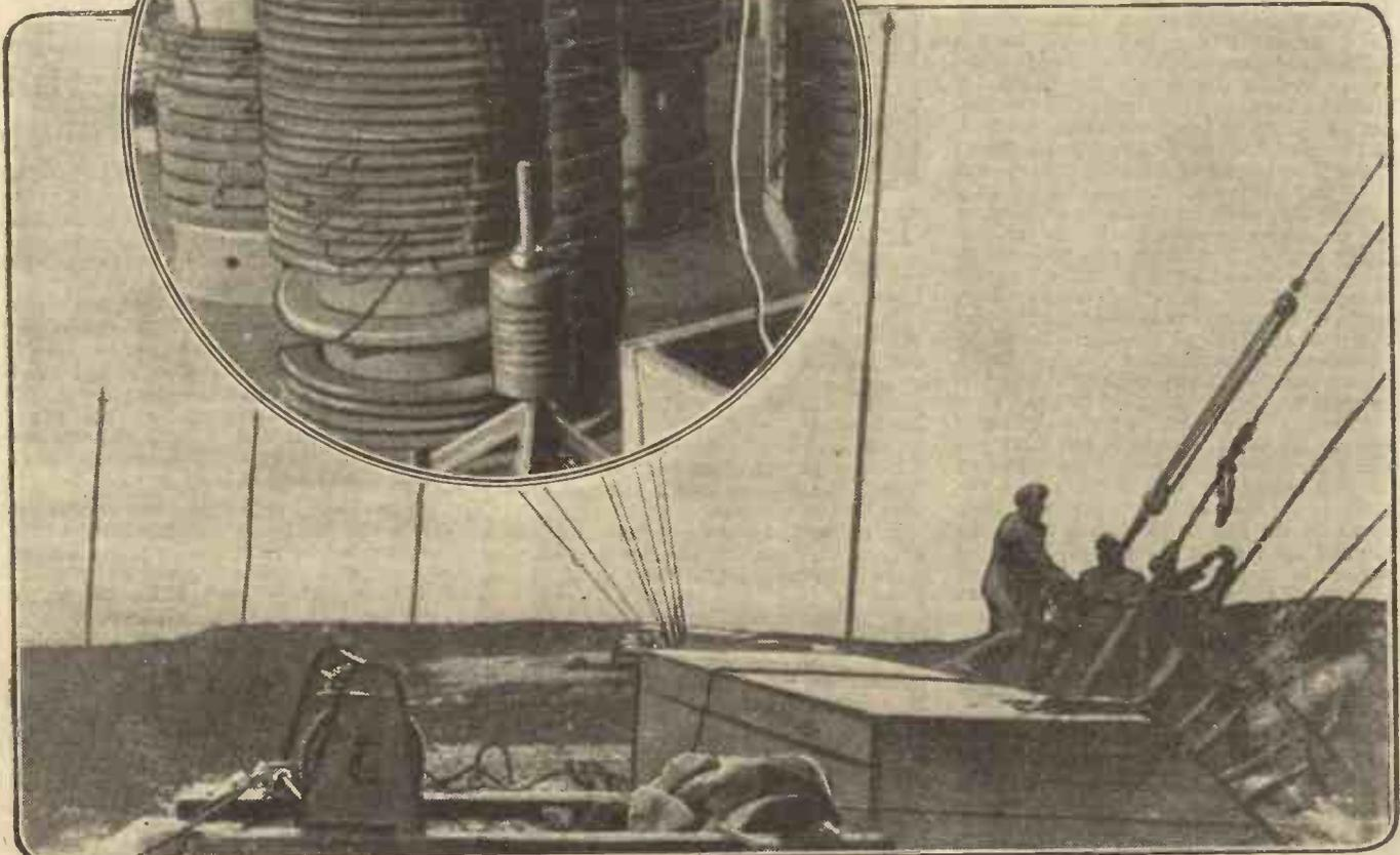
Our photograph in the circle above shows the choke coils used in connection with the old "spark" transmitter. Below, the photograph shows some of the ten steel masts, each 400 feet high, which support the aerial system. The gny ropes are anchored to massive 100-ton concrete blocks and are capable of withstanding an enormous strain.
