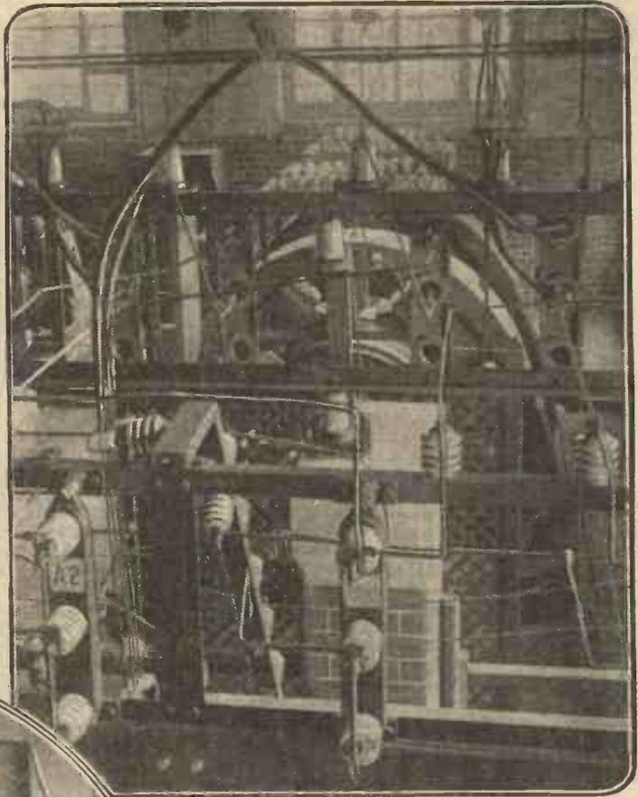
The Marconi Transmitter bank of 56 valves. The action of this type of transmitter is noiseless, and is far more efficient than the old "spark" method of transmission.
