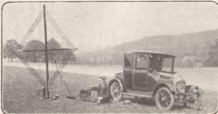
A Motor Car Frame Aerial Set. The frame is in sections and can be quickly dismantled.
