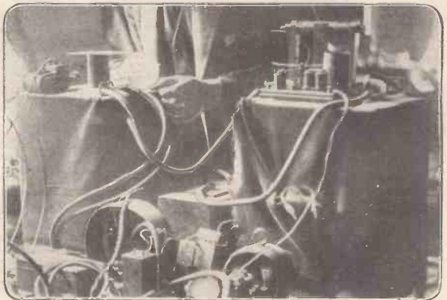
Portion of the Televisor by which the possibility of seeing by wireless has been demonstrated.
