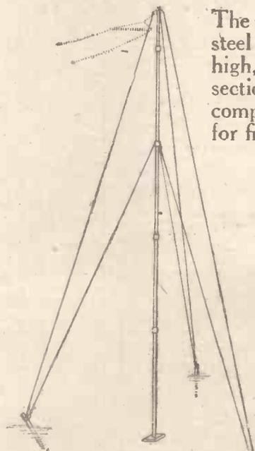
The Chelsea hollow steel mast stands 30 ft. high, is built in four sections, and is sold completely equipped for fixing.
