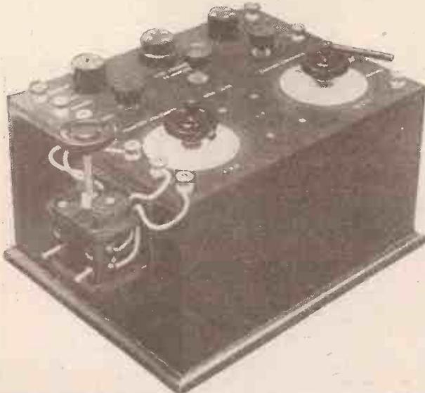
This photograph of the completed Reflex Unidyne Receiver shows the layout of the main components and the relative positions of the tuning controls.
