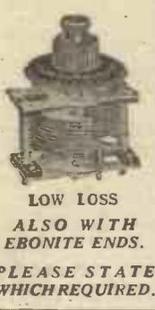
Pig-tail connection to rotor gives silent working. Special Spring top Bush gives a firm but easy movement. Including knob and dial as sketch With vernier. 0003 .. 7/11 0005 .. 8/6 Including knob and dial. No vernier. 0003 .. 5/11 0005 .. 6/6 With geared dial, 12-1 ratio, 6/- each extra. POST 6d. PER SET.
