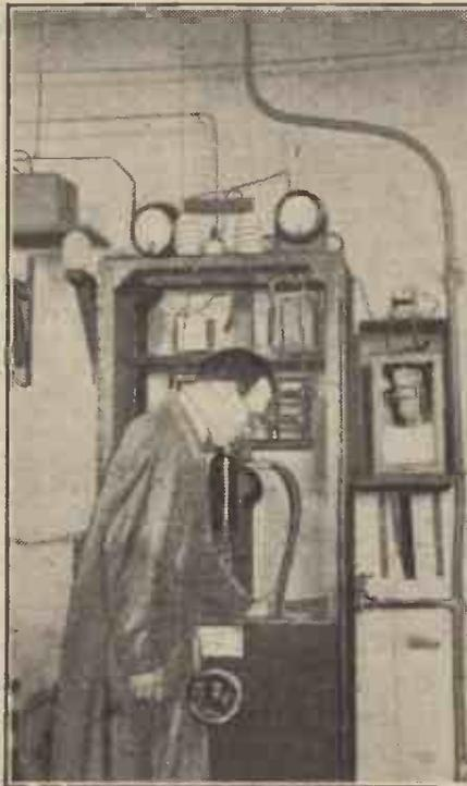
Testing one of the water-cooled valves employed by Radio-Paris, the well-known broadcasting station.
