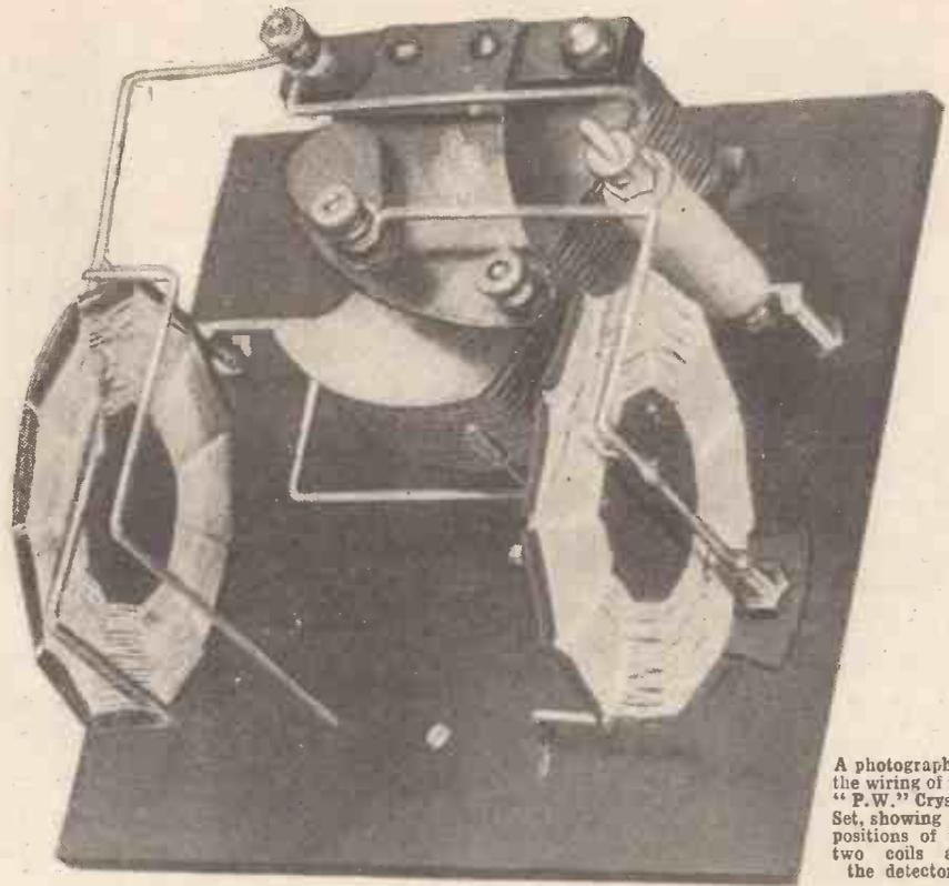
A photograph of the wiring of the "P.W." Crystal Set, showing the positions of the two coils and the detector.
