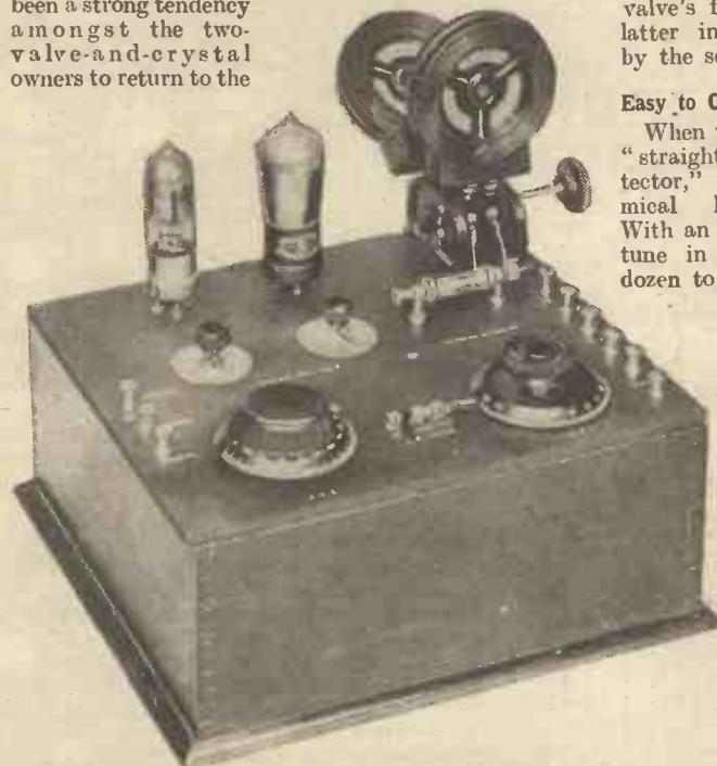
The complete set, ready for connecting up. With the switch as shown, the low-frequency valve is not in use.
