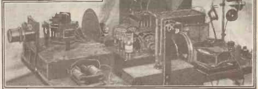
An experimental television transmitter constructed in accordance with Mihaly's system.
