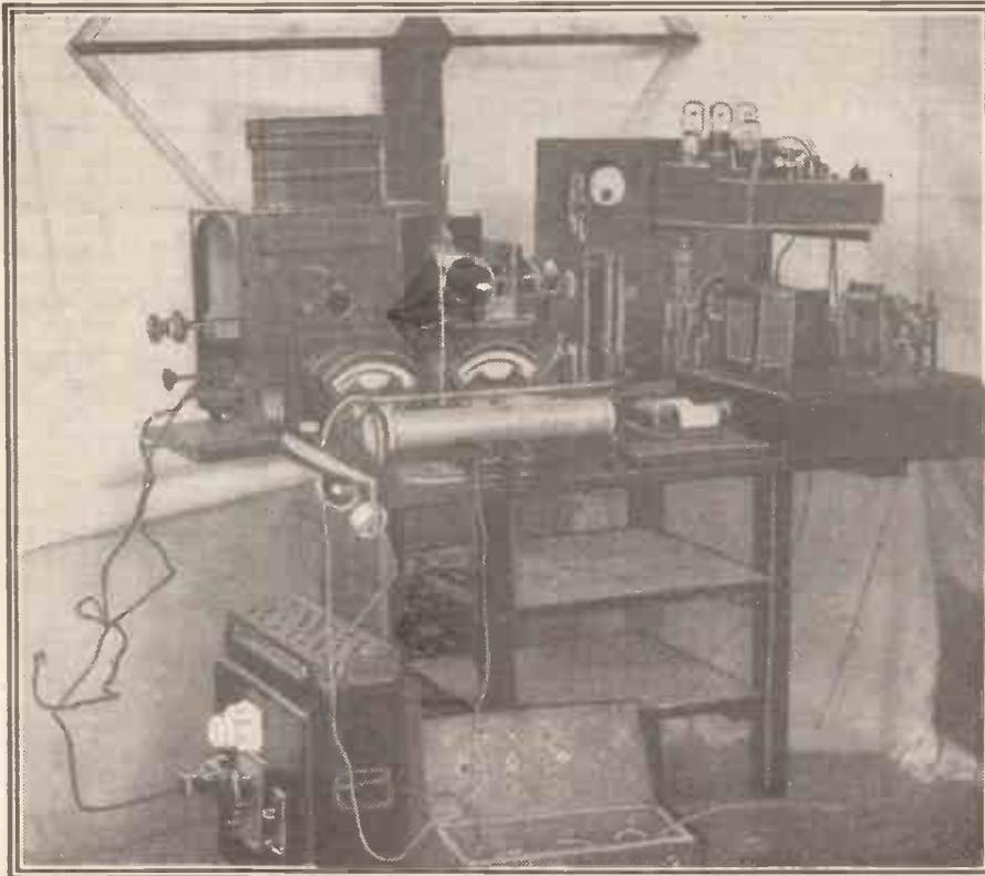
The receiving section of Mihály's experimental television apparatus.
