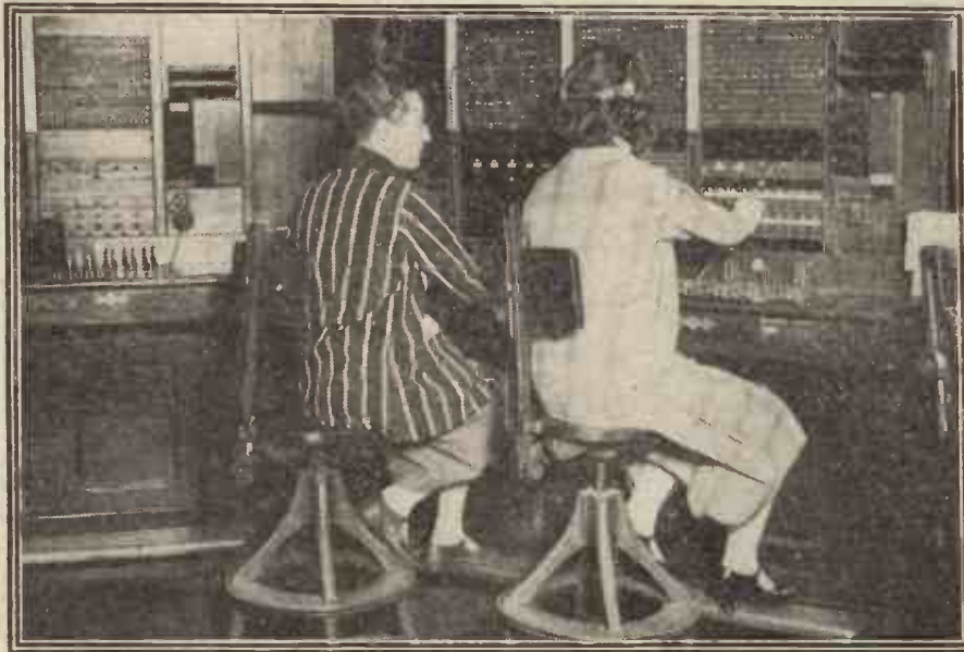
Two of the specially trained telephone girls at the London Trunk Exchange at which English subscribers can be plugged straight through to New York.
