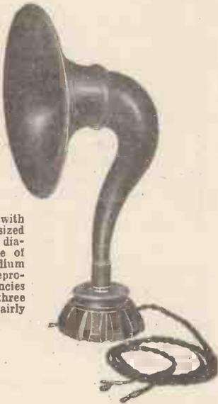
A loud speaker with a medium-sized horn and diaphragm capable of handling medium inputs and of reproducing frequencies above two or three hundred fairly faithfully.
